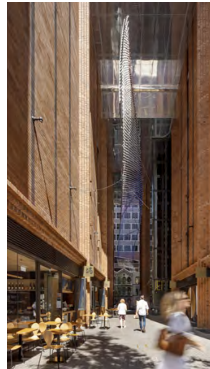
Throughsite link from Clarence Street, showing the bands of dark brick on façade.
