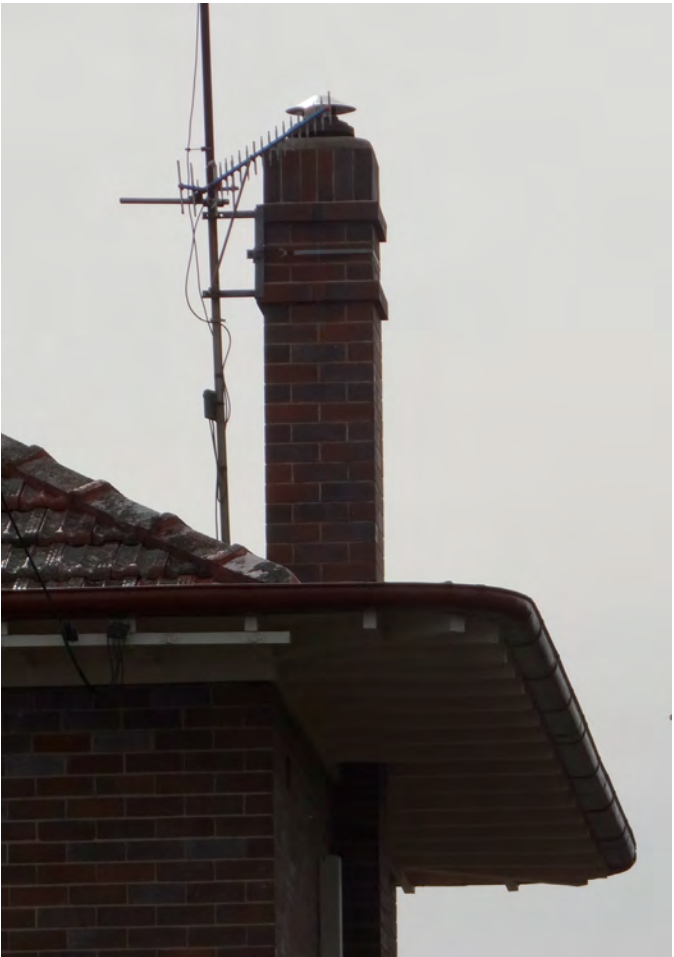
Yet another interesting roofscape - very wide bracketed eaves, perhaps a direct response to the rather harsh climatic conditions
