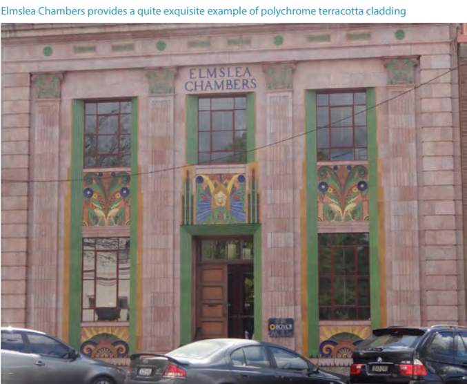
Elmslea Chambers provides a quite exquisite example of polychrome terracotta cladding
